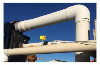
Scrubber biogas flow meter; measures biogas leaving scrubber (biogas + air injection).
