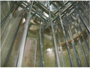
First deck of bioreactor looking up towards second deck (without packing material) – vertical PVC piping for feeding bacteria and rinsing packing material.
