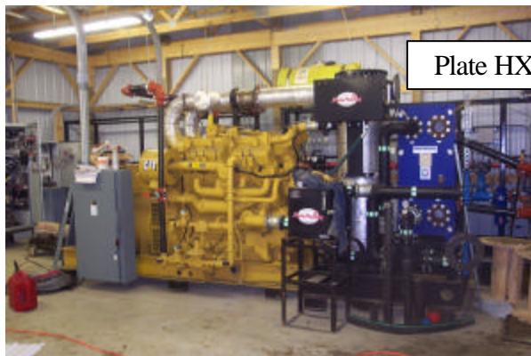
Partially Installed Engine Skid at Emerling
