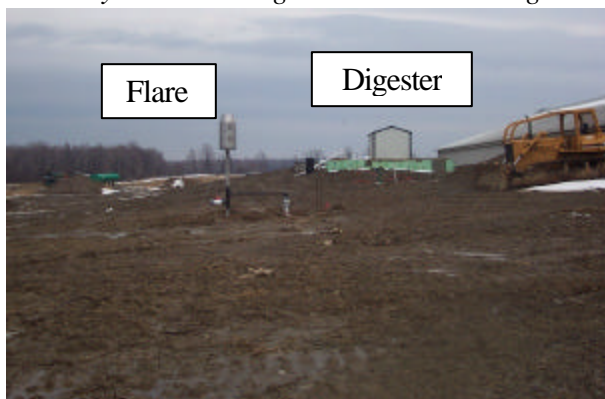
Digester and Biogas Flare at Sunny Knoll
