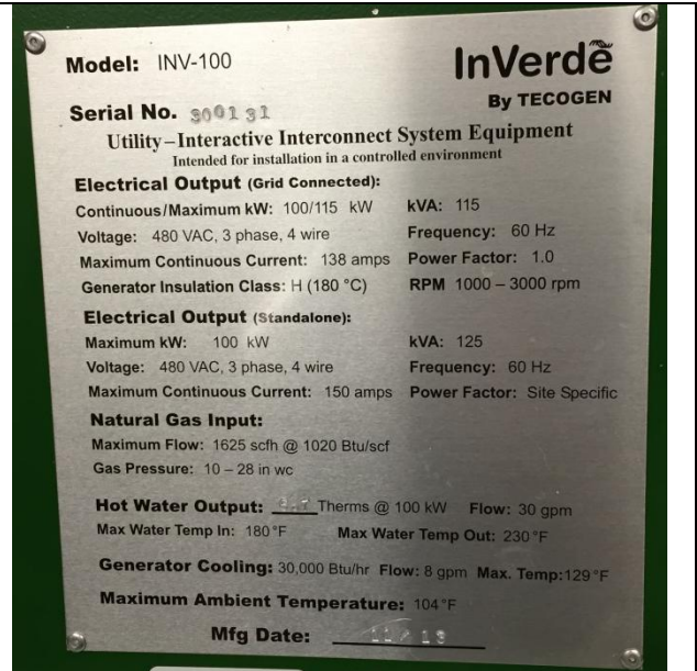
Nameplate for 231 Steuben Street
