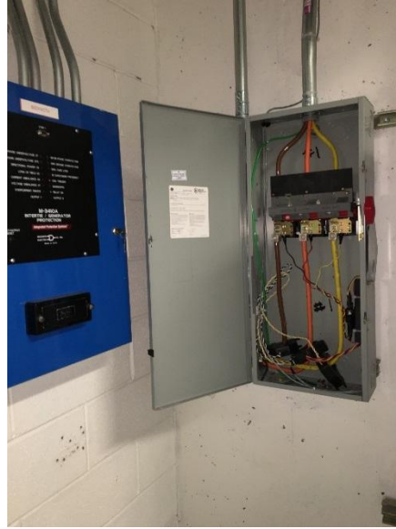
Generator 1 Power Transducer
