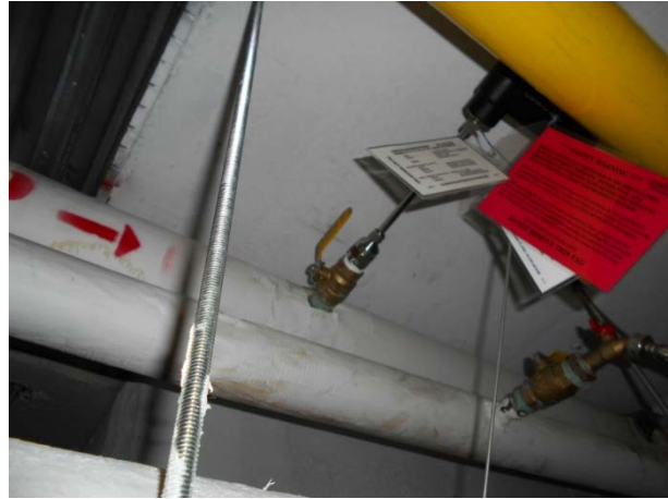
Onicon F-1100 insertion flow meter
