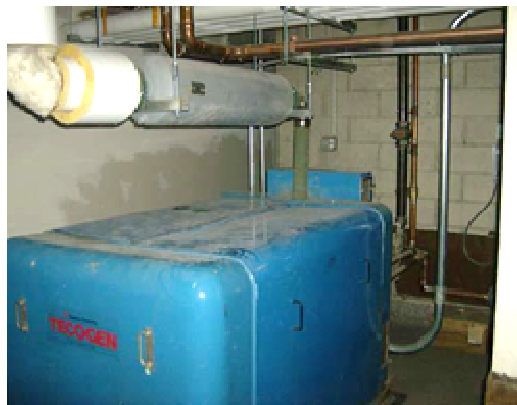
FIGURE 3 SINGLE CHP MODULE SHOWN DURING INSTALLATION
