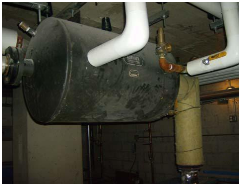
FIGURE 5 EXHAUST HEAT RECOVERY HEAT EXCHANGER
