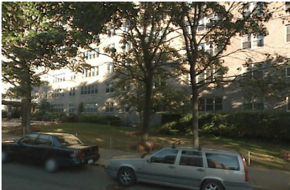
FIGURE 2 RIVER POINT TOWERS, BRONX, NEW YORK
