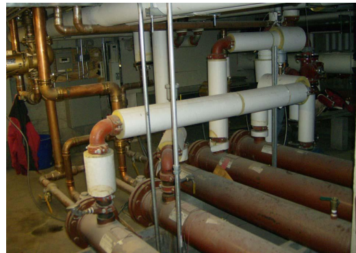
FIGURE 6 HEAT EXCHANGER NETWORK SERVING END USES
