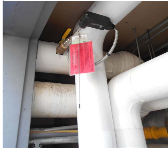
Un-commissioned Square D Ion 7550 parasitic power meter.
