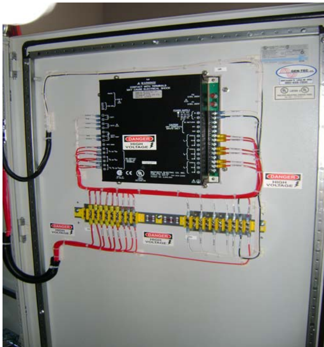
Beckwith Protective Relay (from back of door)
