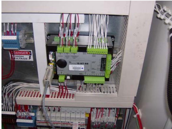
Intelisys NT and output to Carbon Catcher
