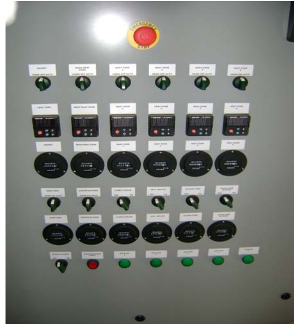
Digester Control Panel (from GHD)
