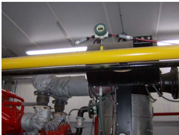
FGE – Sage flow meter, measuring gas to engine.
