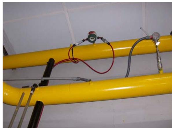
FGF – Sage flow meter, measuring gas to flare
