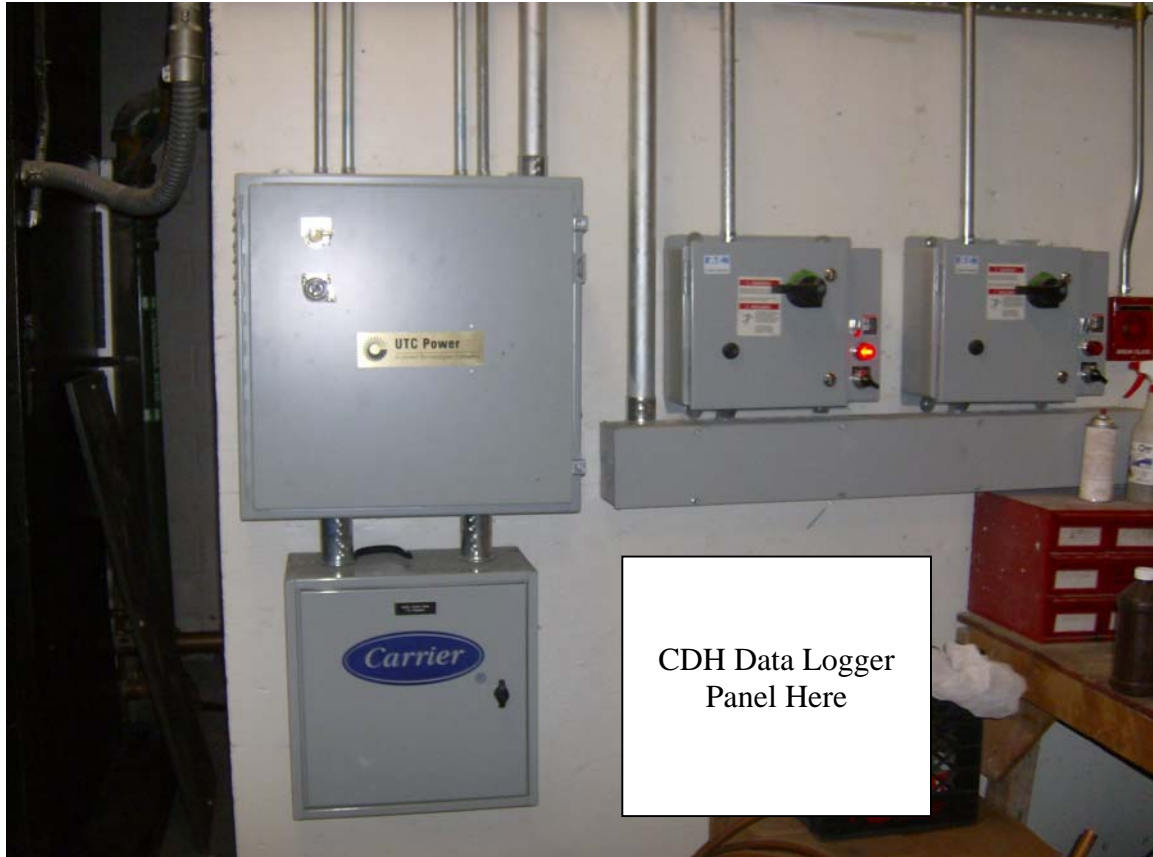
Figure 12. Existing UTC Power RMS Panel and Proposed Data Logger Location
