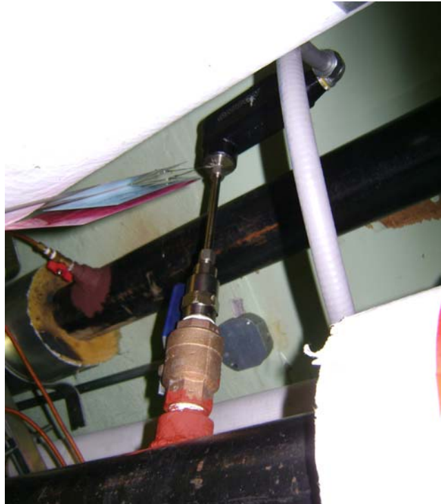
Flow meter on cogen loop (FM-2)
