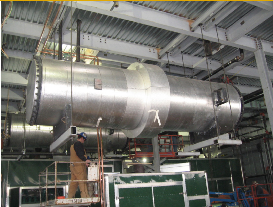
FIGURE 9 HEAT RECOVERY HEAT EXCHANGER INSTALLATIONS
