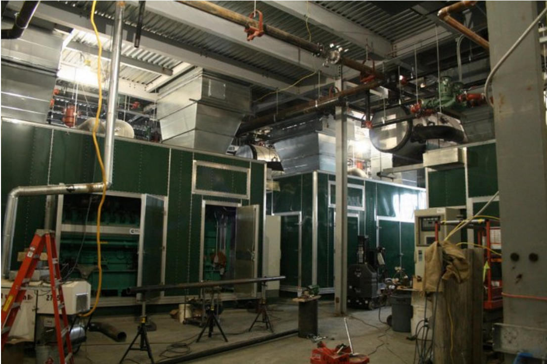
FIGURE 8 ENERGY CENTER UNDER CONSTRUCTION
