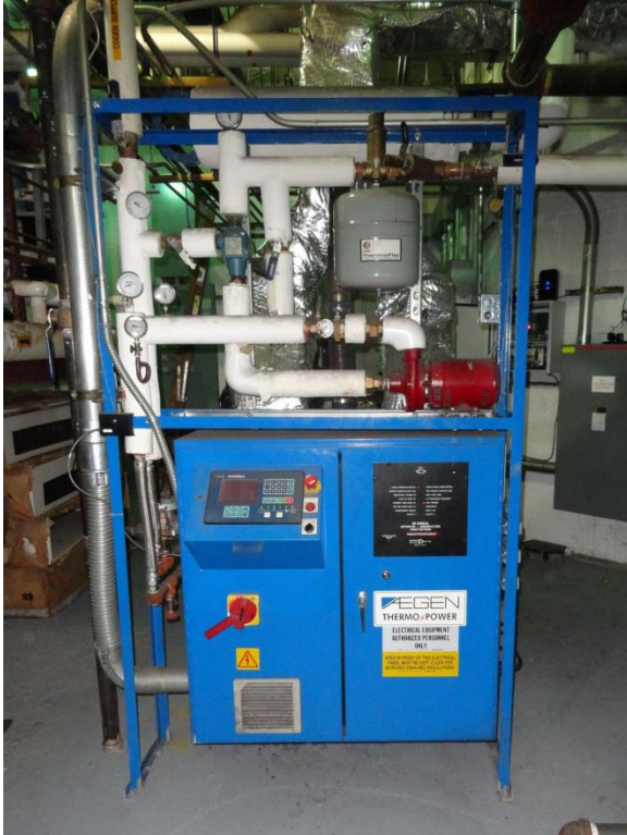
AGEN 75-kW Engine Generator
