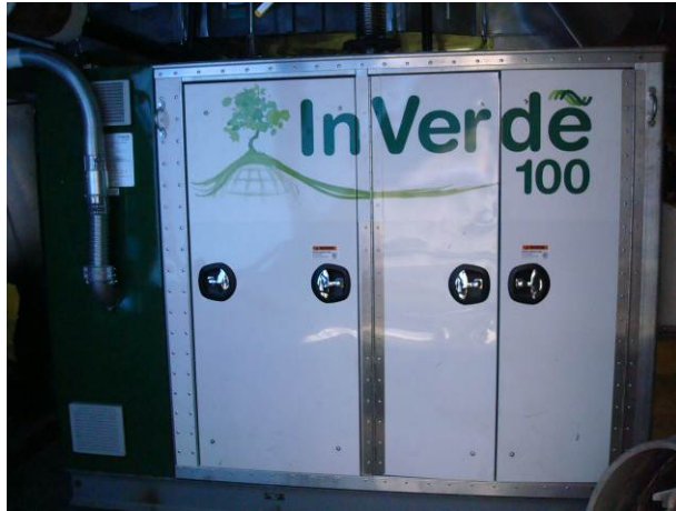
Engine-Generator Enclosure
